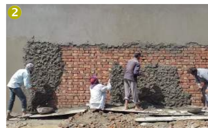
▲ Renovation of the boundary walls
